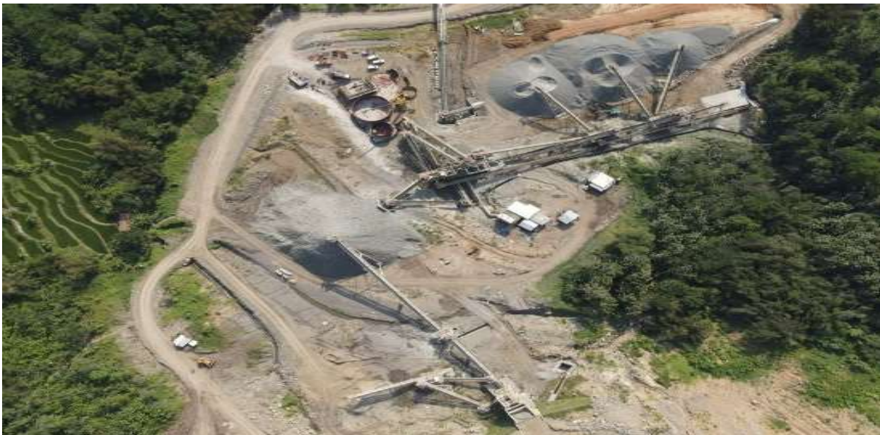
Crusher & Washing Plant Area
